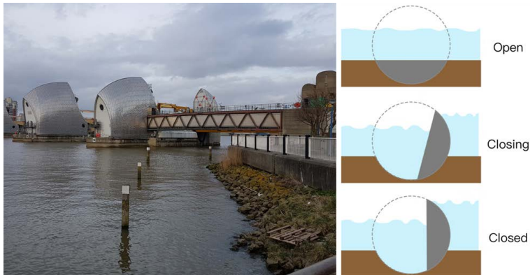
Fig 5 Sluice in River Thames, England and its operation Source: Kleon3
