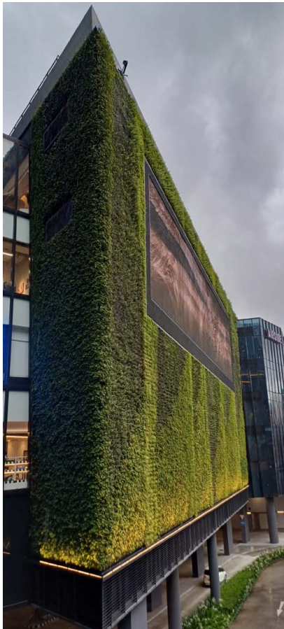
Fig 1 Building with vertical greening
