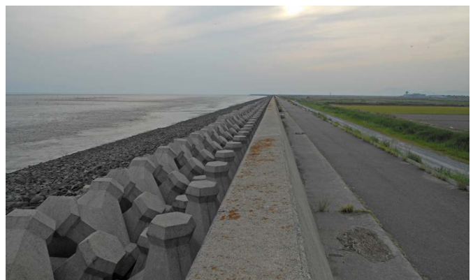
Fig 4 Coastal protection structures in Japan Source: Pekachu
