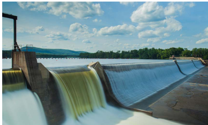
Fig 3 Hydro-electric dam Source: American Public Power Association
